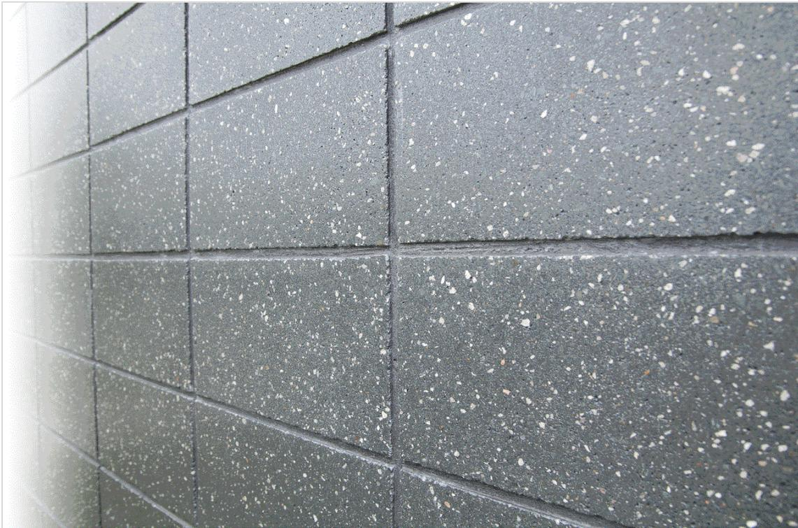
*A clear coating weather seal provides a matt finish to this wall and helps prevent efflorescence.*
