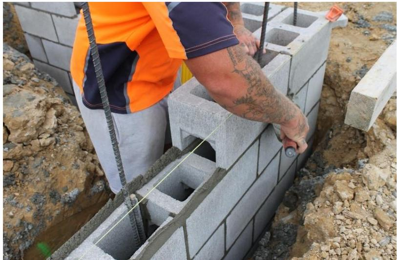
Laying of masonry units shall be in accordance with NZS 4210. All masonry units shall be laid in mortar in courses, true to line, plumb, and level to the tolerances of NZS 4210, unless otherwise specified.
